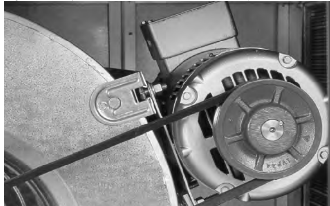
Figure 1: Adjustable Motor Mount and Pulley
