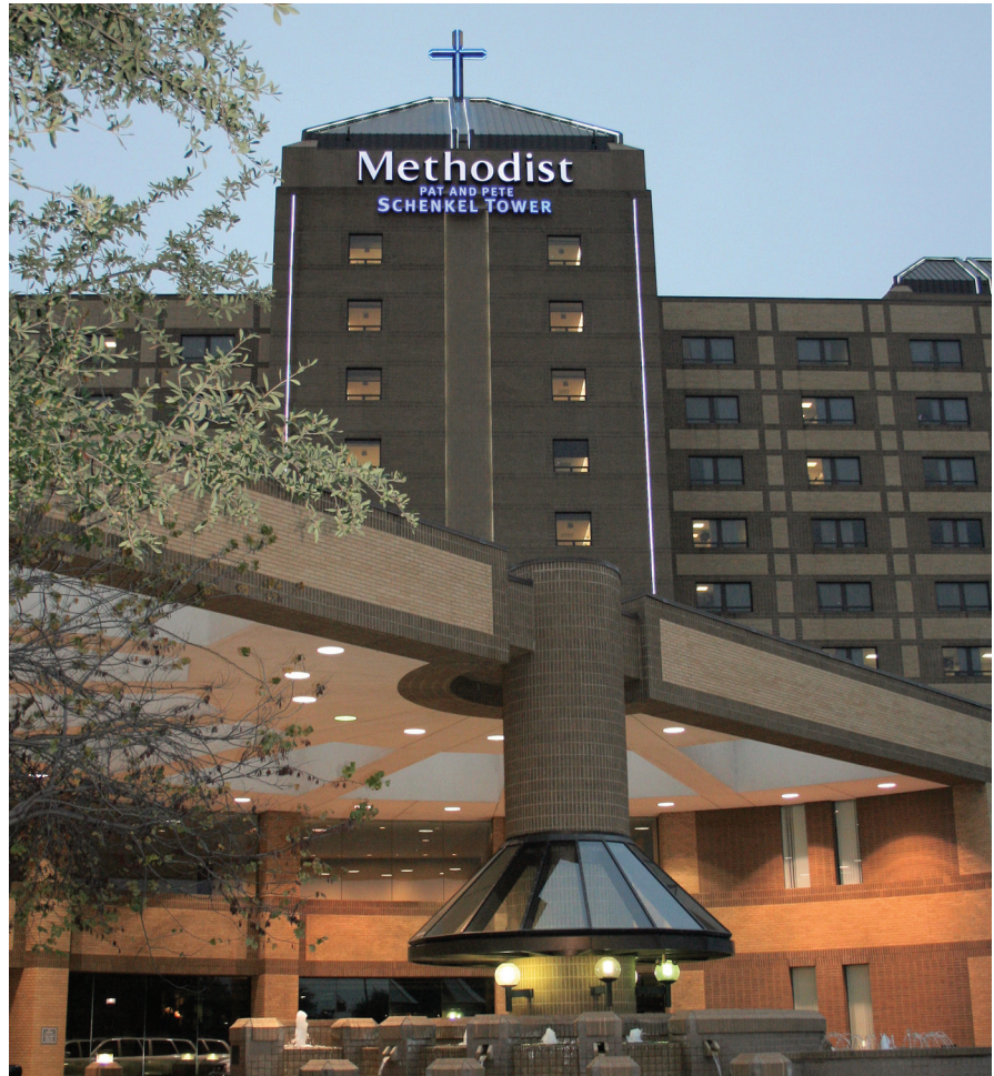
Methodist Dallas Medical Center achieved an 18-month payback on a new HVAC system that includes a 2,000-ton McQuay dual-compressor centrifugal chiller.
