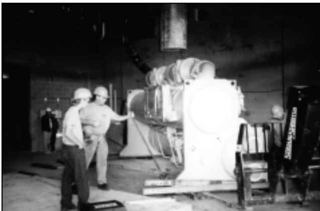
McQuay chiller installation at Tampa Stadium.
